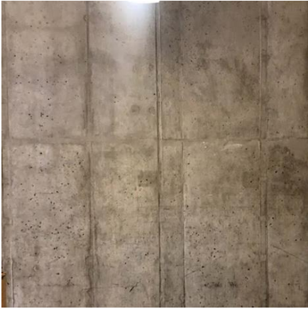
Concrete – Smooth (Interior)
