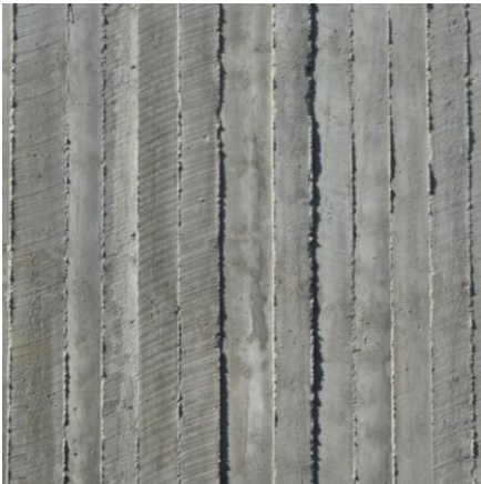
Concrete – Board Form
