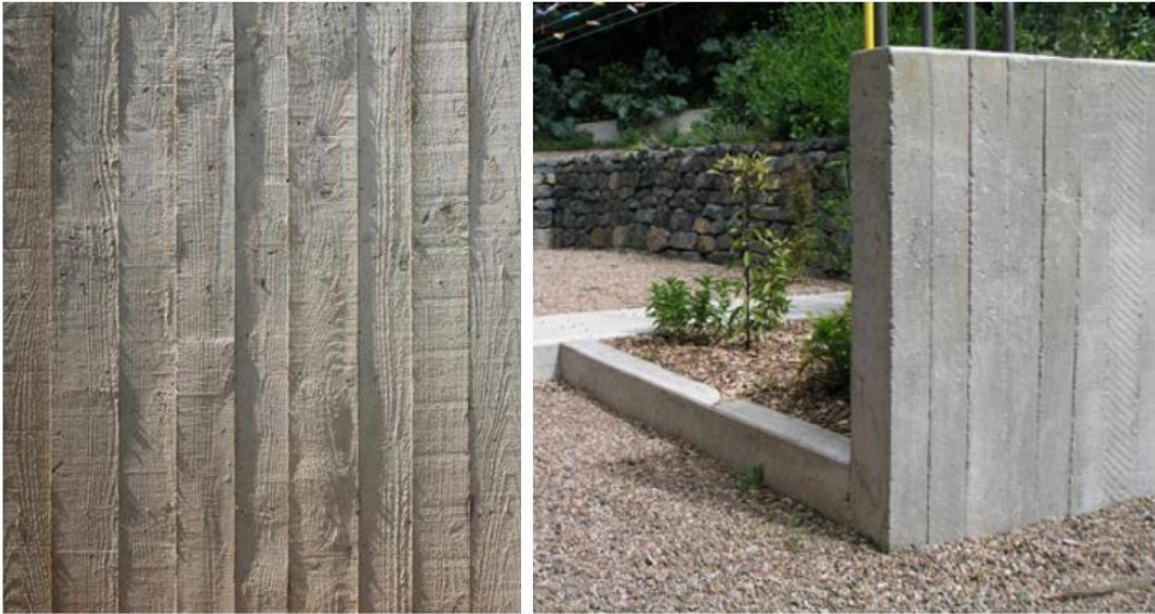
BOARDFORM CONCRETE WALLS
