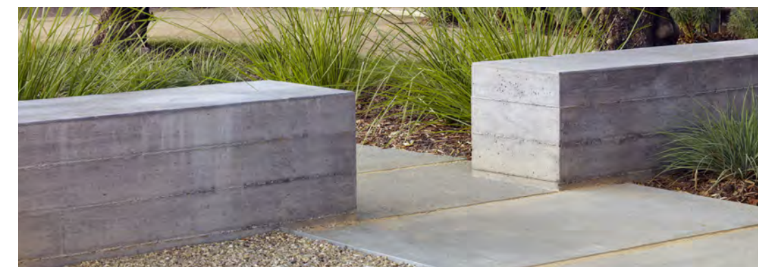
BOARD FORM CONCRETE BENCH
