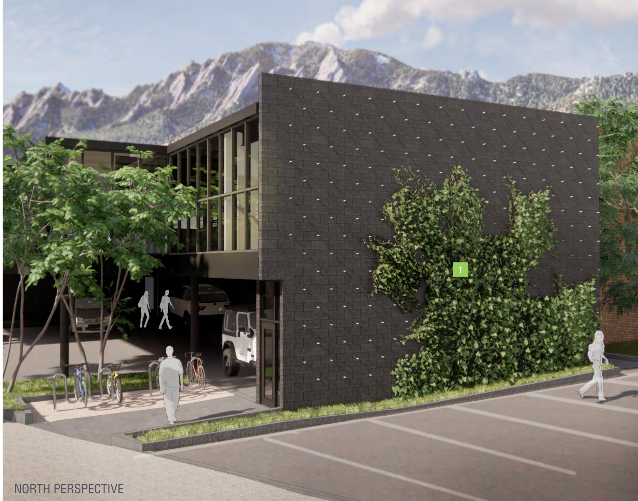
1 STEEL CABLE TRELLIS GREEN WALL
