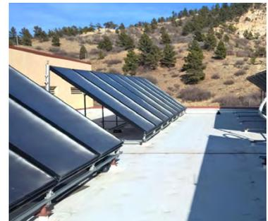
A solar thermal system on the roof of the UCCS Recreation Center provides more than half the energy required to heat the swimming pool and spa. On sunny days it provides 100 percent of the energy, offsetting the use of natural gas.
