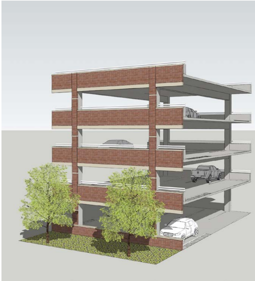
Brick Veneer Precast System
