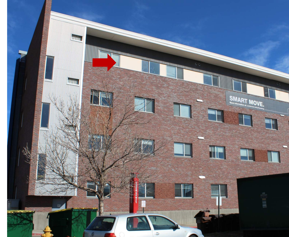
Cement board panels at east elevation
