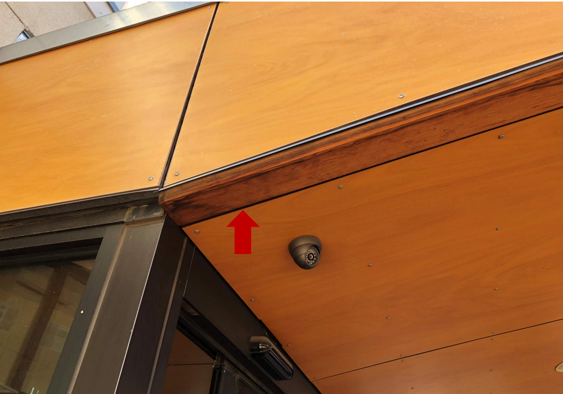
Potential replacement of weathered wood trim at courtyard canopy
